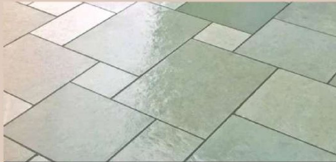
KOTA FLOORING IN EACH GALA / UNIT
